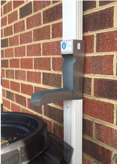
Rainwater diverters are used to direct rainwater from the downspout into your rain barrel.
