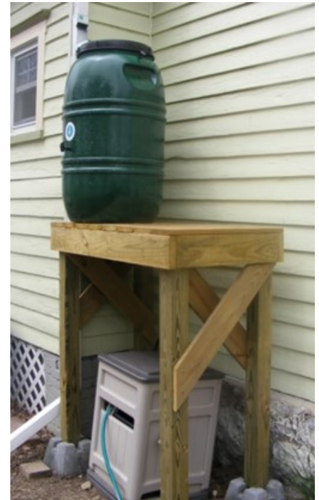
Elevating your rain barrel will increase your water pressure.
